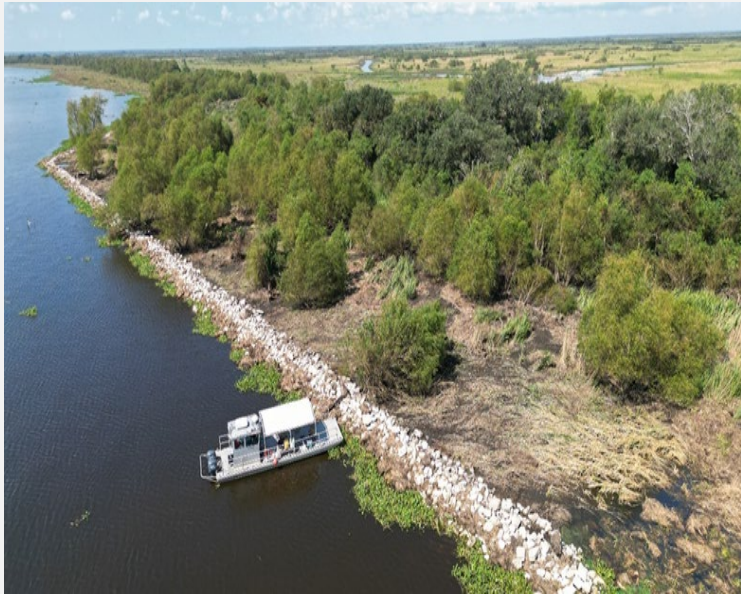
*Aerial view of a successful shoreline protection project on the western shoreline of Lake Salvador. (BA-0015-X2)
