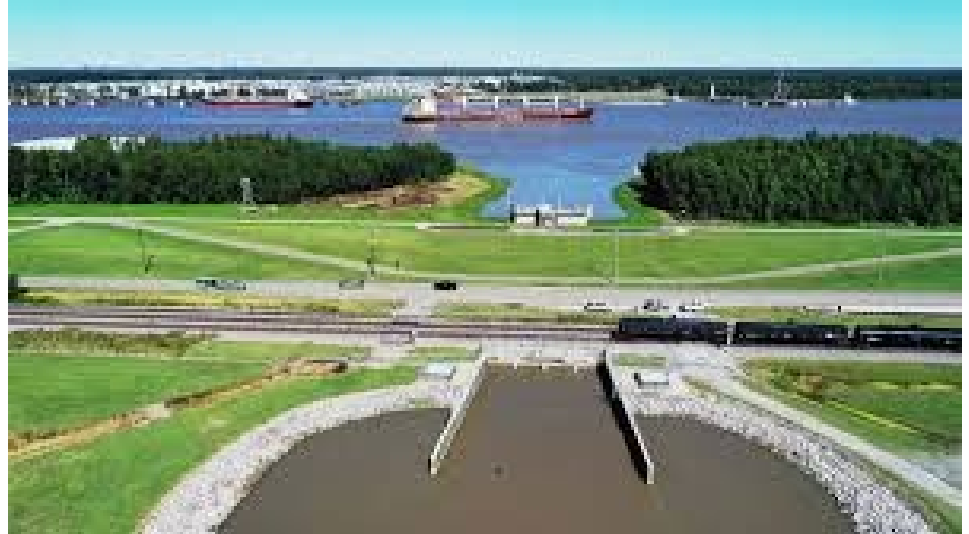
*Davis Pond Freshwater and sediment diversion
